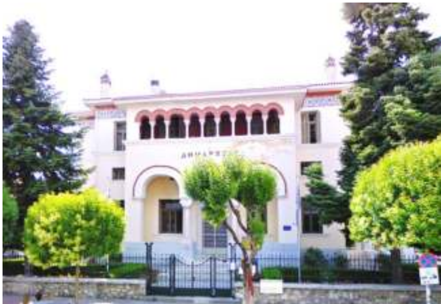
Figure 22 External view of the City Hall building
