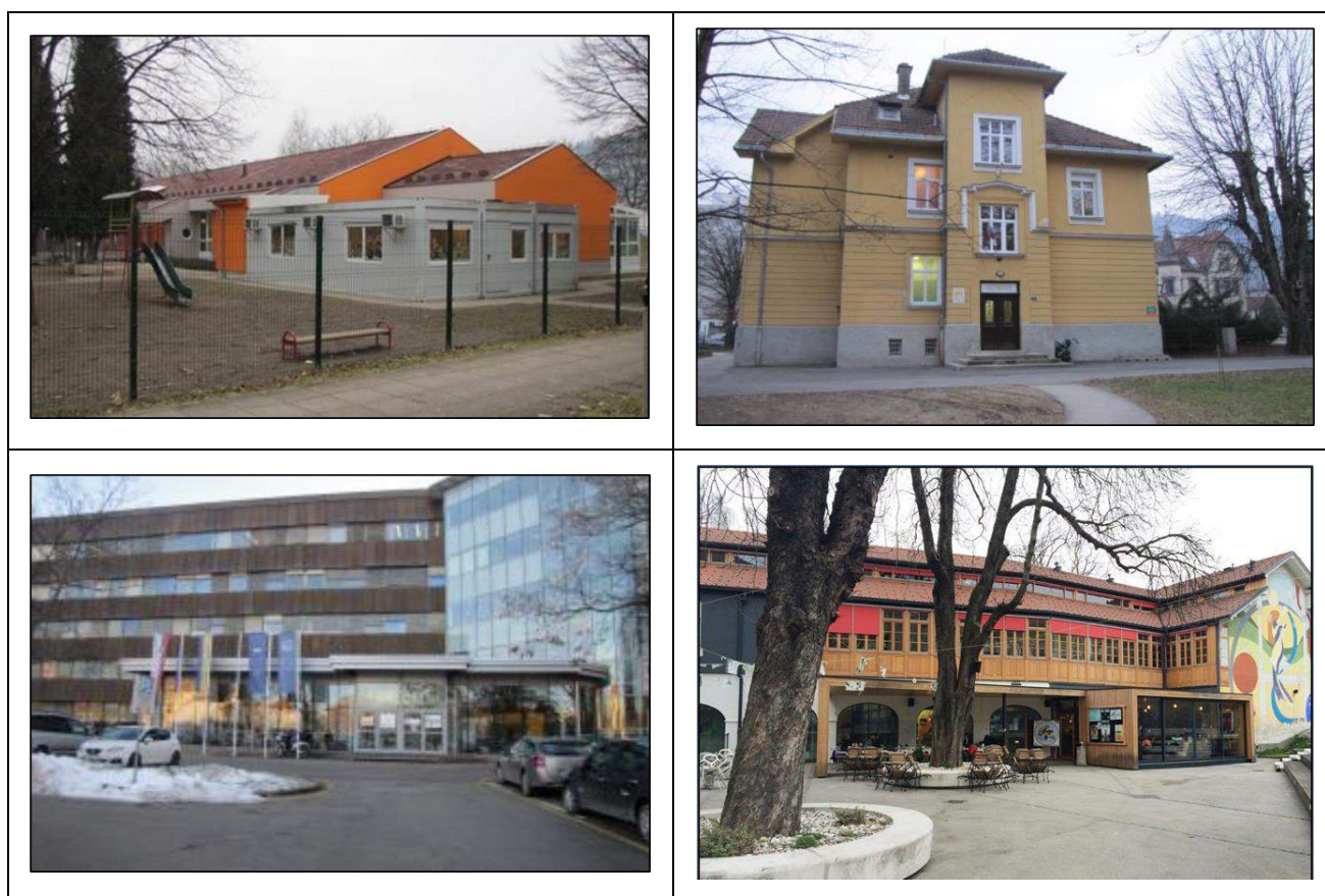
Figure 9: The case-study buildings in “Glazija and Otok”: Kindergarten Luna (top left), Kindergarten Sonce (top right), Faculty and office building at Mariborska ulica 7 (bottom left), Celje Youth centre - CMLC (bottom right).
