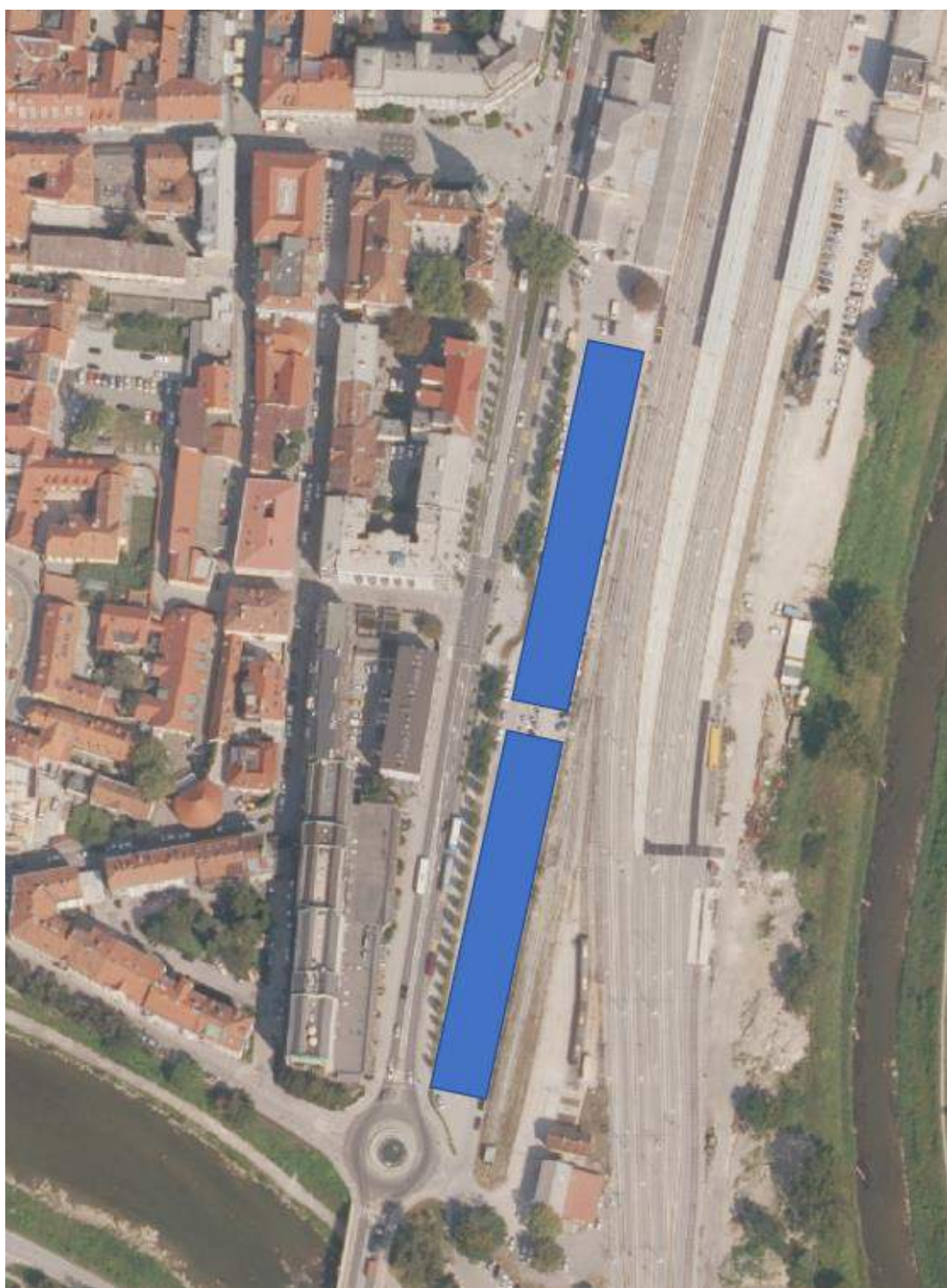
Figure 13: Parking lot “Railway Station” in replication area PED 1 “Old City” - a site considered for installation of PV canopies
