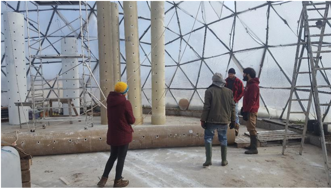
Figure 7 Raising aeroponic pipes inside the Dome (photo by author, March 2018)
