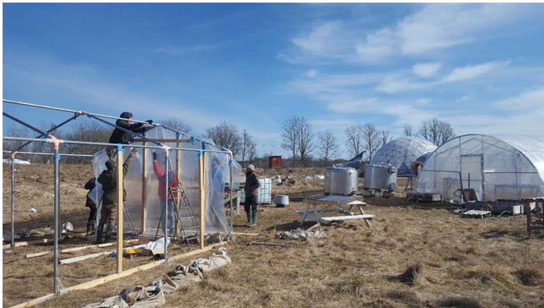
Figure 6 Construction of the greenhouse "Pépita" with the dome, polytunnel, and horseshoe nr. 1 visible in the background (photo by author, March 2018)
